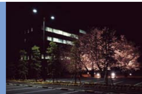
街路灯 Street Light
